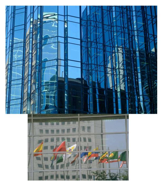
\*Note the irregularly shaped flags and trees have less noticeable distortion to their reflective image than the linear lines of the building.
