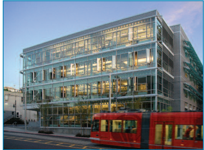
New Solarban 72 Starphire glass is comparable to Solarban 70XL glass, pictured here on AIA COTE award winner, The Terry Thomas in Seattle, with significantly better visible light transmittance and similar solar control.
